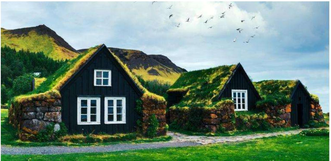
If you happened to visit Iceland, you may remember the characteristic houses with green roofs. This original cover is made of turf, a compact combination of grass and legumes. The houses consist of a stone
